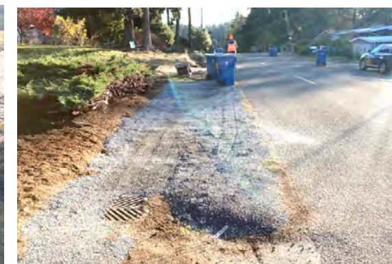
The neighborhood has many gravel ROW areas.
