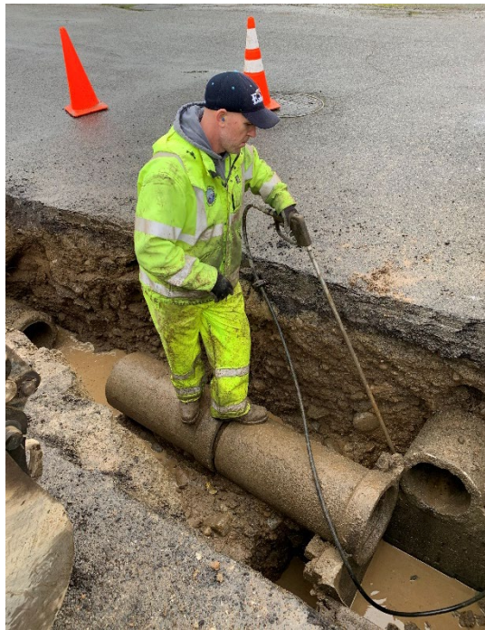
Crews work to replace damaged storm pipes.
