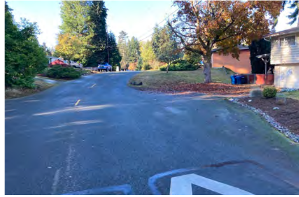
Section of 191st St SW with excess pavement that could be removed and retrofitted with bioretention.
